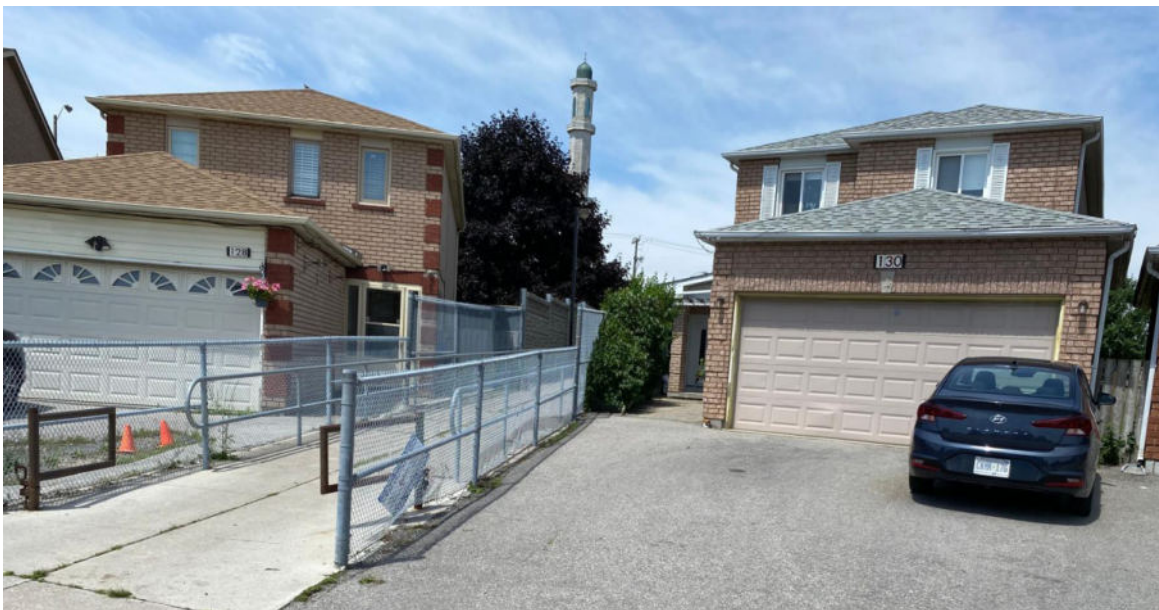
The Two Houses On Robbinstone Drive Scarborough
