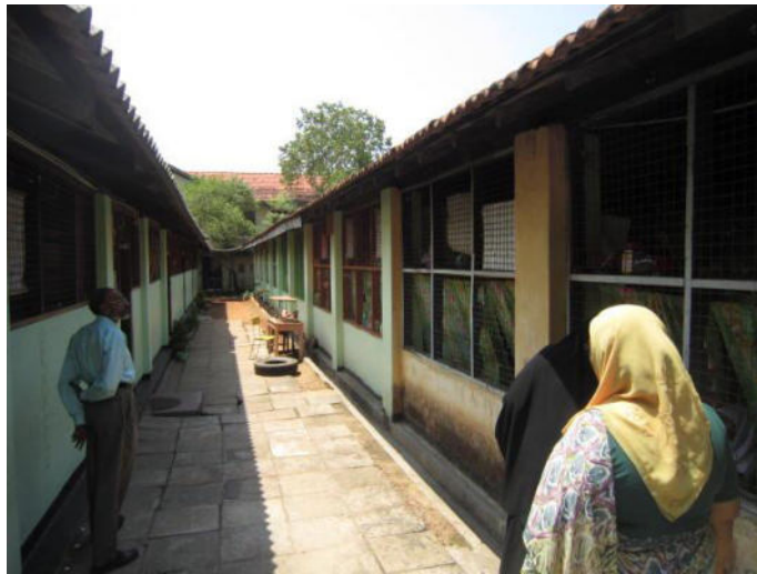
THE PRINCIPAL SHOWING THE STATUS OF THE BUILDING
