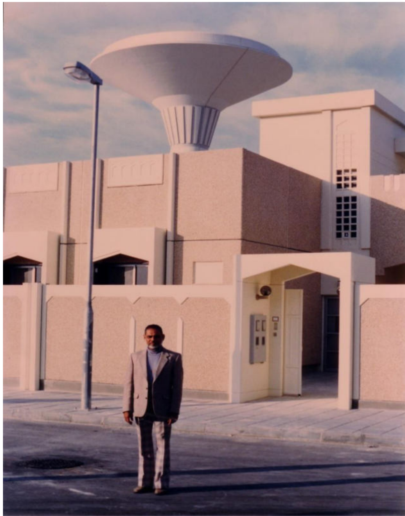
HOUSING PROJECT IN QATIF SAUDI ARABIA
