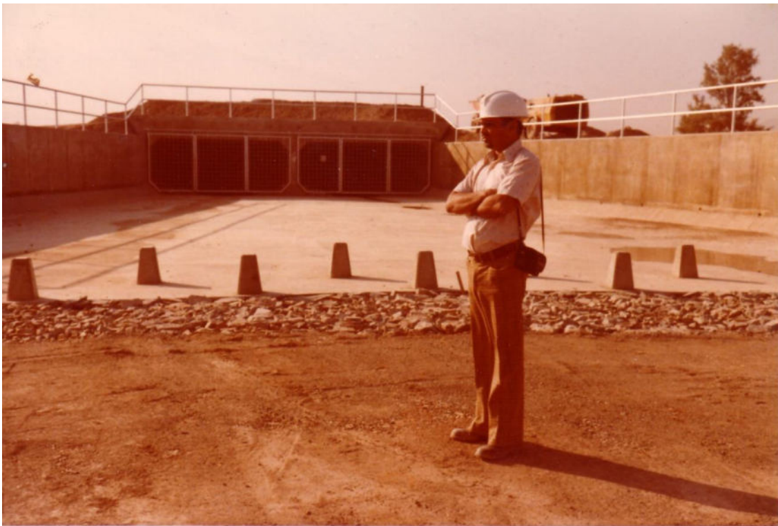
ADMIRING THE COMPLETED OUTFALL OF MEDINA STORM DRAINAGE SYSTEM, BEFORE LEAVING TO RIYADH IN DECEMBER 1979.
