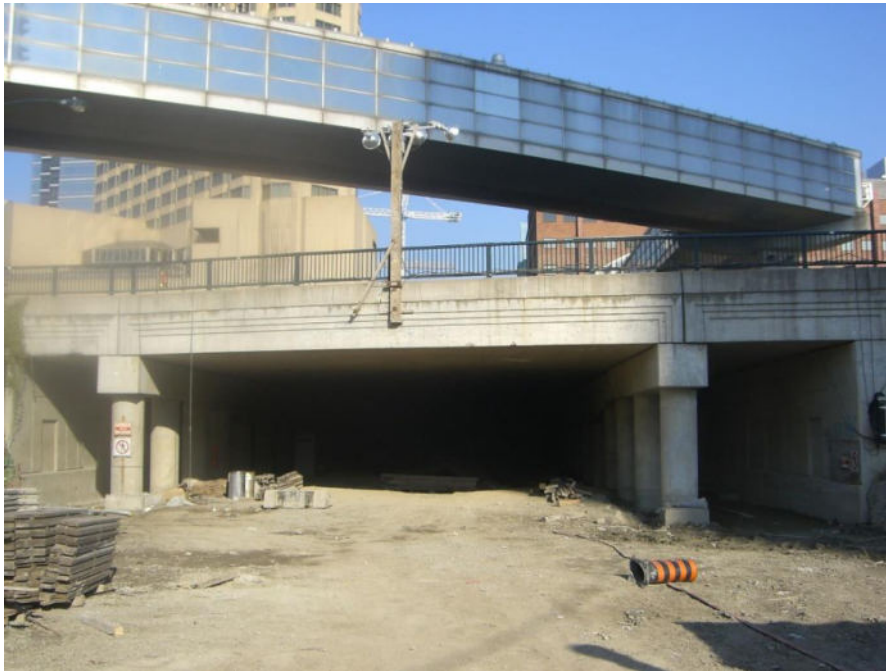
THE SIMCOE STREET TUNNEL, USING PRE-CAST GIRDERS
