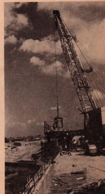
ROMA FLYER on retaining wall work.
