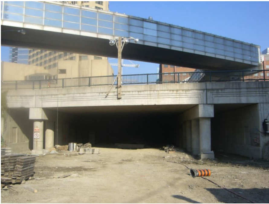
THE SIMCOE STREET TUNNEL, USING PRE-CAST GIRDERS
