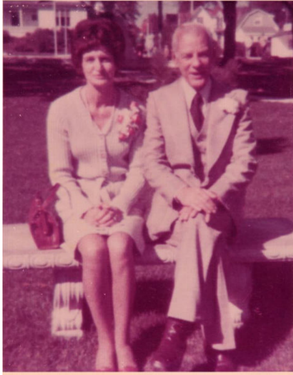
AGA'S FIRST CONTACT IN PITTS CONSTRUCTION GEORGE & BETTY
