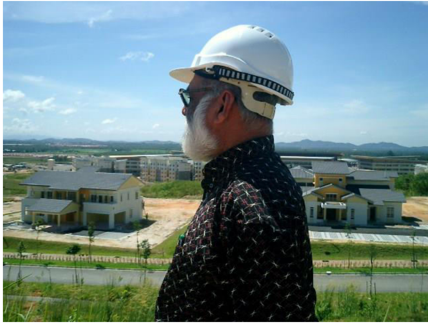
THE LAST LOOK AT THE AIMST UNVERSITY BEING BUILT AT ALOR ESTAR MALAYSIA. IT IS ALMOST 85% COMPLETE. PICTURE TAKEN IN NOVEMBER 2004.
