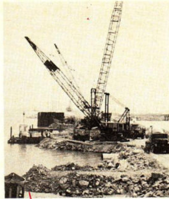
VIEW is south from shore. Footings for pier are placed from causeway.
