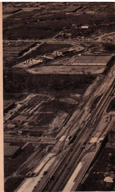
DETOUR maintains four lanes of traffic
