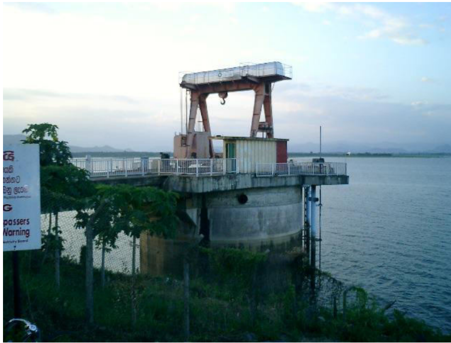
RIGHT BANK POWER PLANT AT UDAWALAWE PROJECT. PICTURE TAKEN IN JANUARY 2005.
