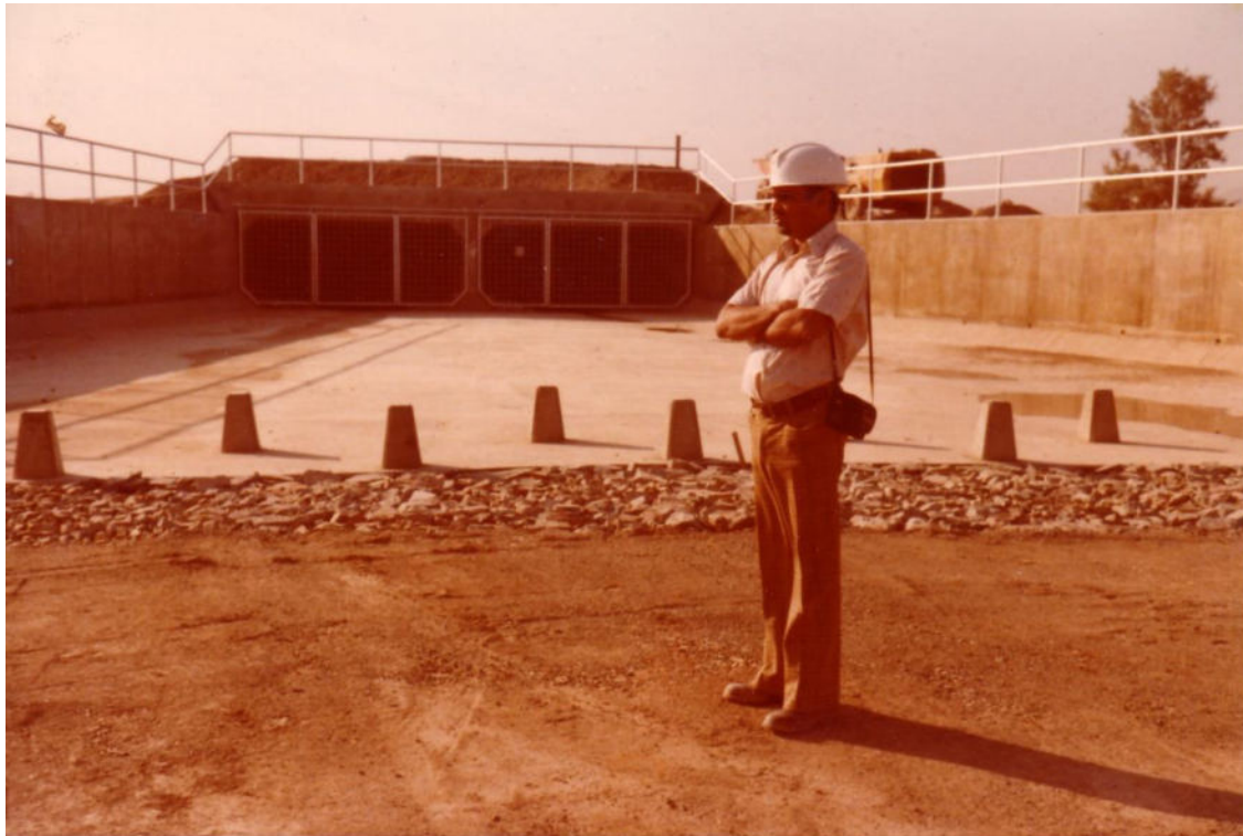
ADMIRING THE COMPLETED OUTFALL OF MEDINA STORM DRAINAGE SYSTEM, BEFORE LEAVING TO RIYADH IN DECEMBER 1979.
